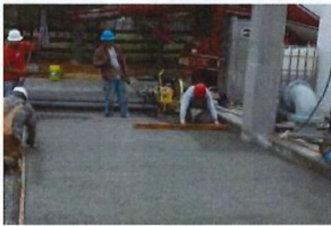
Pervious concrete – during placement
